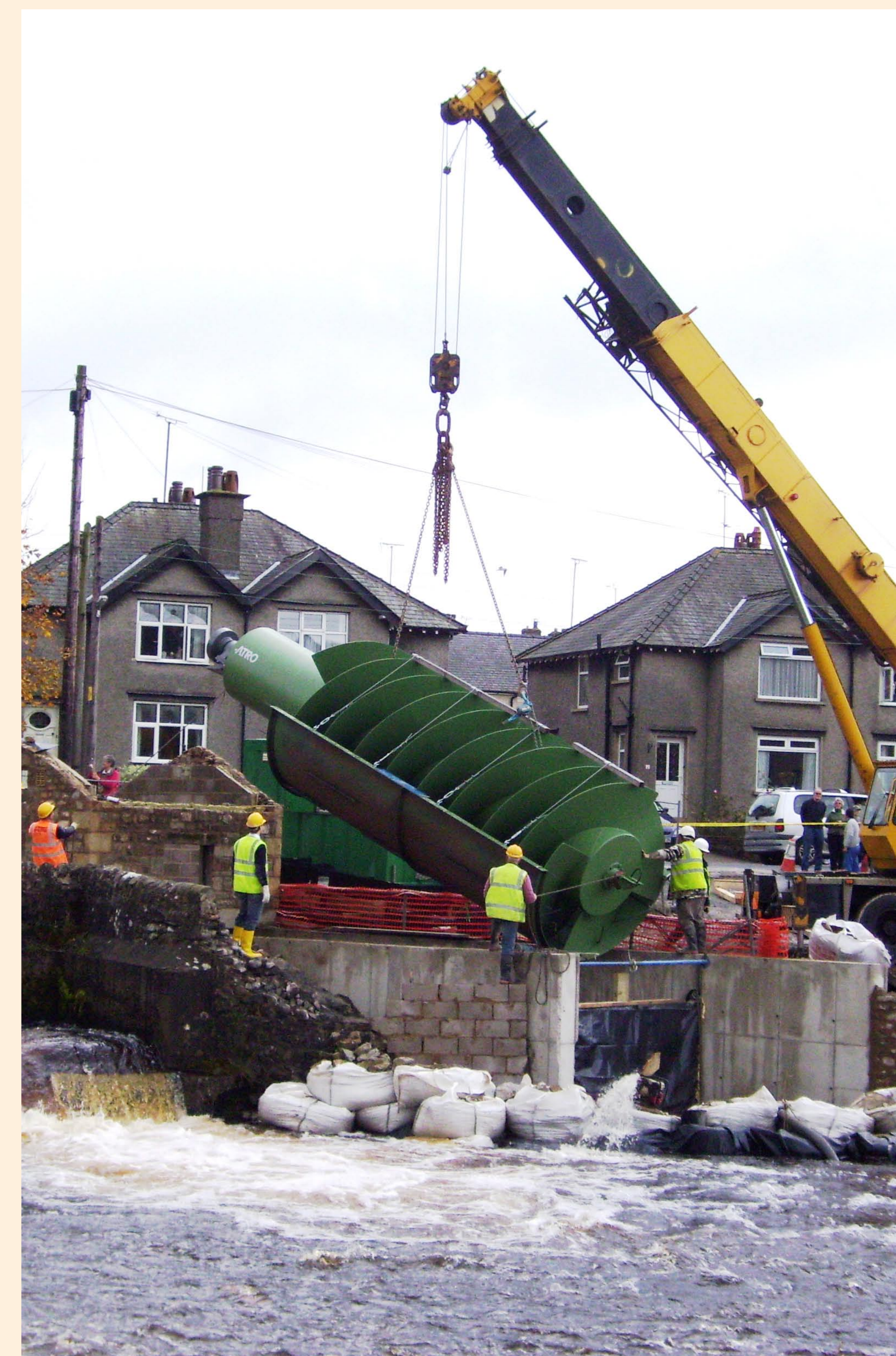
▲ Delivering the Archimedean screw to site Courtesy of Settle Hydro
